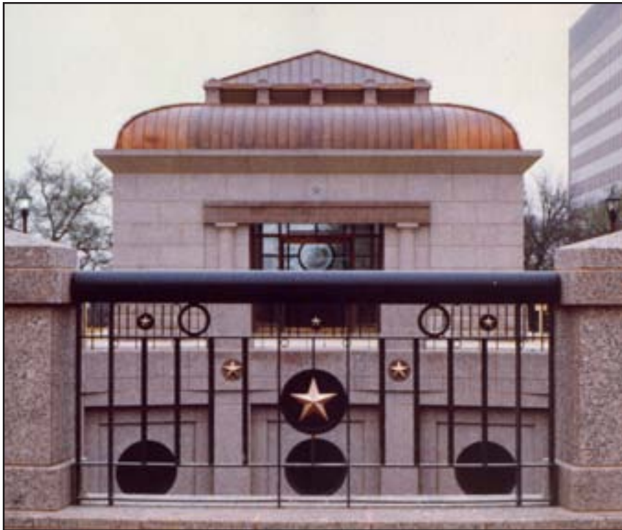
Photo courtesy of State Preservation Board, Austin, Texas. Photographer Griff Smith.
