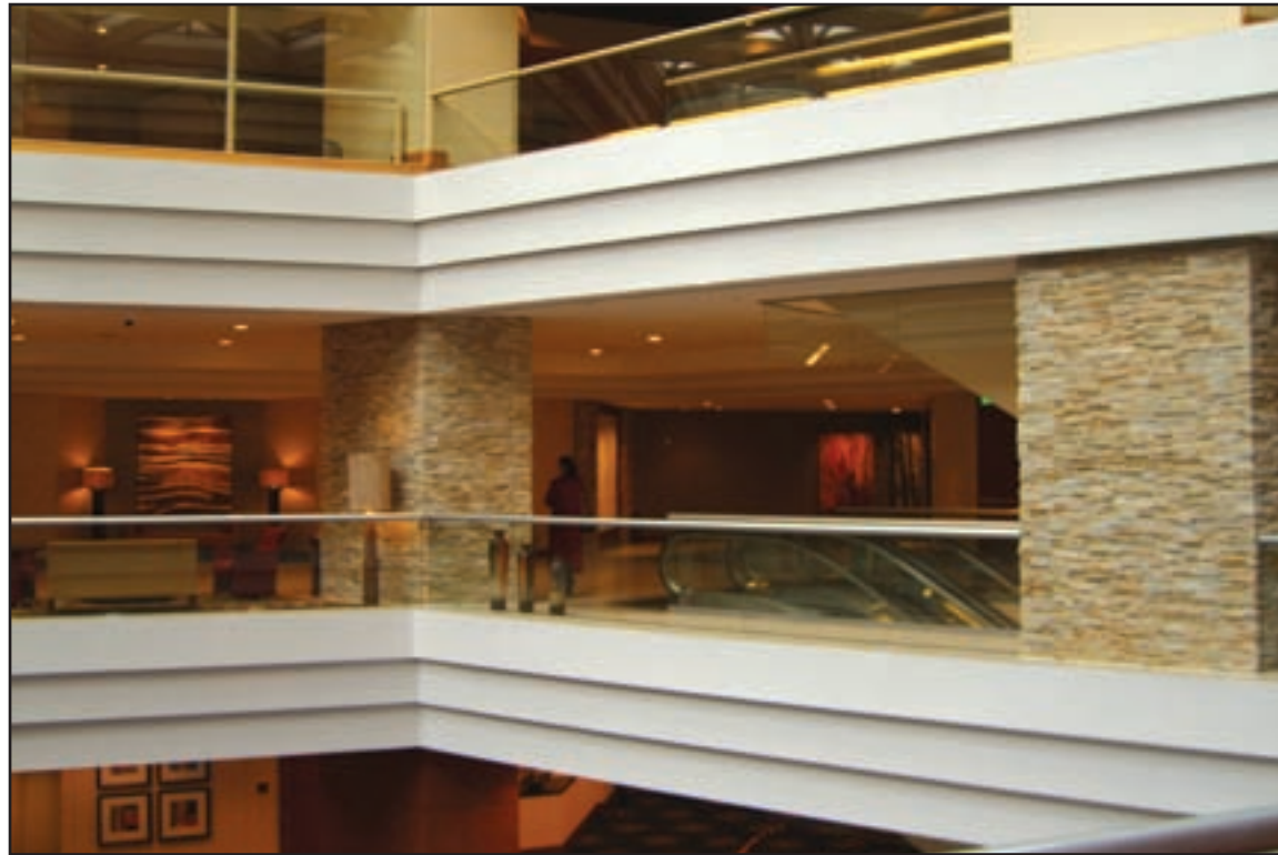
RIGHT: Columns at the Marriott are clad in Sierra Sandstone Shadowstone.
