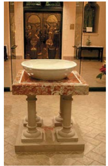
Marble from the original altar and sandstone from a landscape retaining wall were used to create cladding and columns for the new baptismal font and altar at St. Anne's Cathedral in Great Falls, Mont. Stone restoration and photographs by Malisani Inc.
